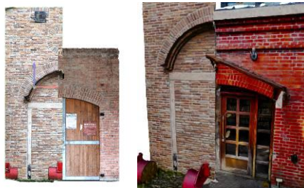
Fig. 4: Examples of reconstructed components and arches of different spatiotemporal backgrounds presenting different curvatures, endings, and numbers of bricklayers.
